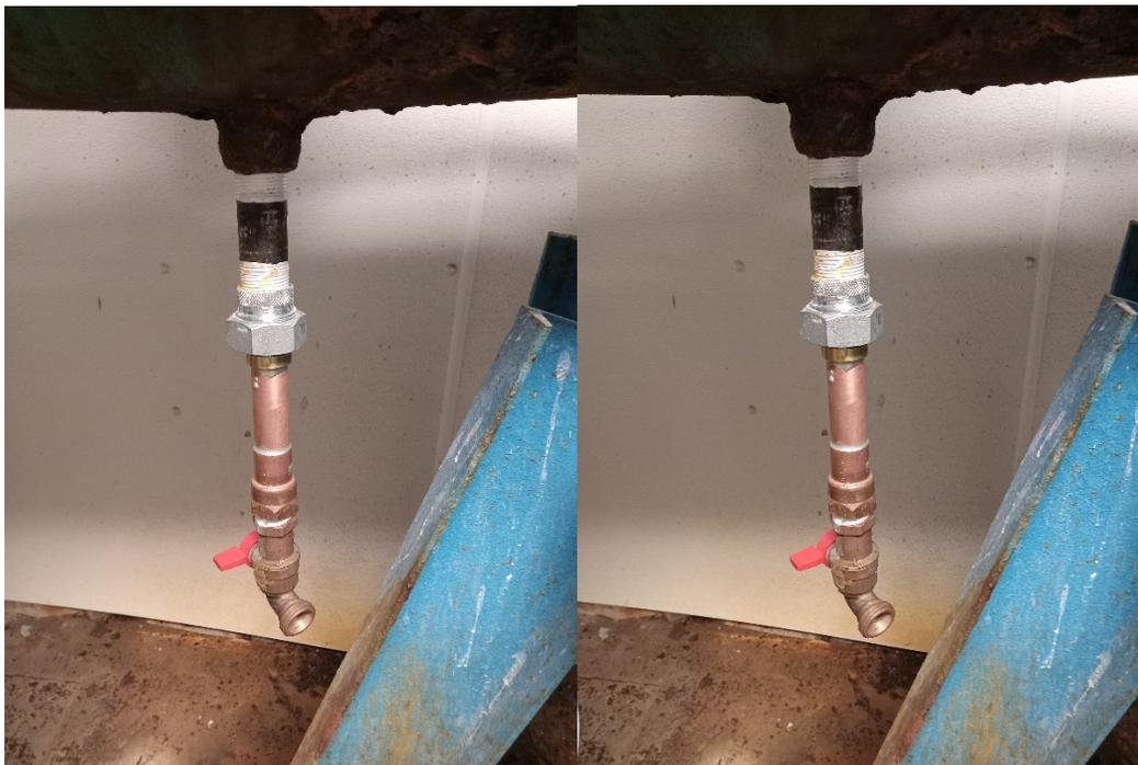
The water treatment plant needs an upgrade and repair. The corrosion from the chlorine and general atmosphere has caused the failure of the emergency repair. This would be a large project to include replacement of all the pipes exposed in the plant as well as the chlorine injection system. The failure of any part of this system will be catastrophic. We have very little components for repairing this system and our other necessary resources would be over strained to complete such a big repair.
